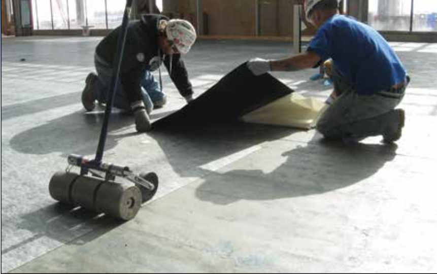
Protecting the floor from substrate movement
